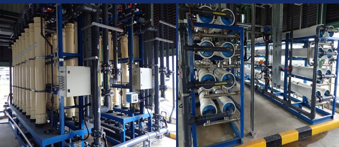
The Microfiltration Pre-treatment System (left) and Reverse Osmosis System (right) work in tandem to treat and recover industrial wastewater for process use
