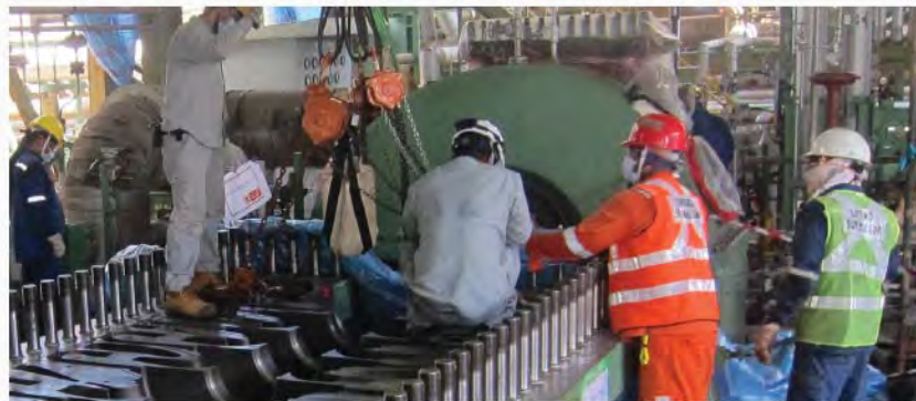
Compressor overhaul work in progress at Compressor house
